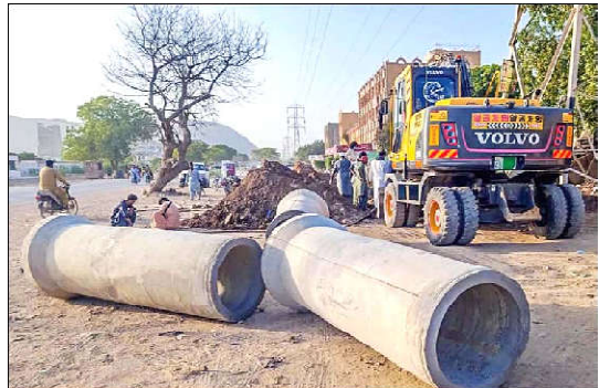
Local government department oversees construction of new sewerage lines in Hub, Pakistan.
