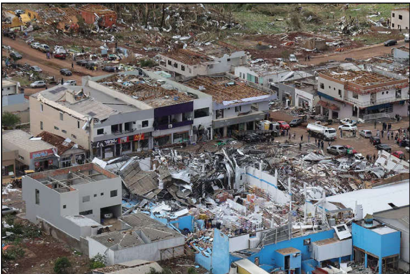
An aerial view shows damaged buildings after a tornado hit Rio Bonito do Iguaçu, Parana state, Brazil.
