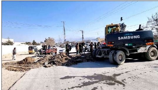
QUETTA: Construction underway for new gas pipelines on Samungi Road in Quetta.
